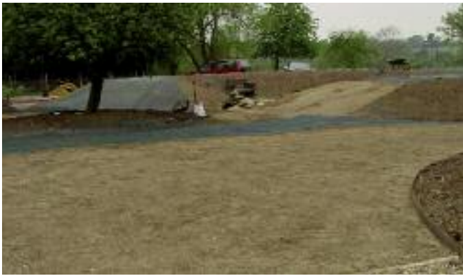
Newly landscaped installation... Green TurfProtecta® laid and covered with a layer of topsoil and seed.
