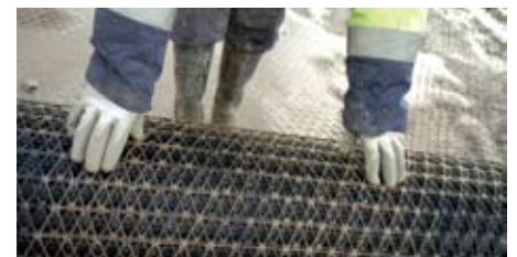
TriAx geogrid unrolled on site.
