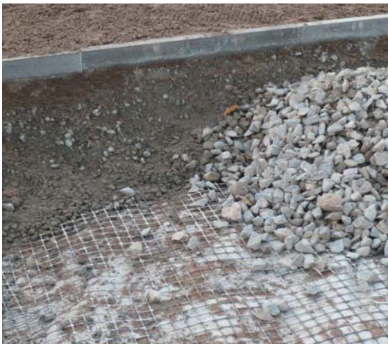
SG20 stabilisation geogrid installed in a road bed construction
