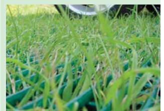
After installation - grass grows through quickly
