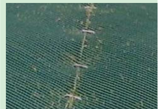
Mesh 'Butt' joined using U-pins
