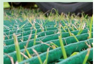
Mesh after installation
