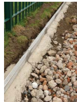
Edging kerbs installed
